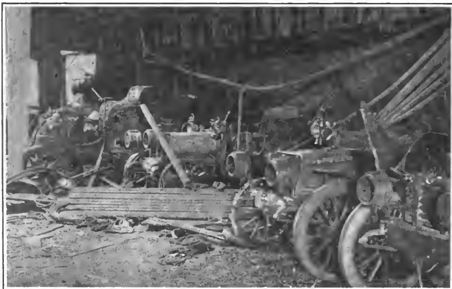
CORNER OF MAIN FLOOR, SHOWING DAMAGE TO DECAUVILLE CARS AND BUILDING.
